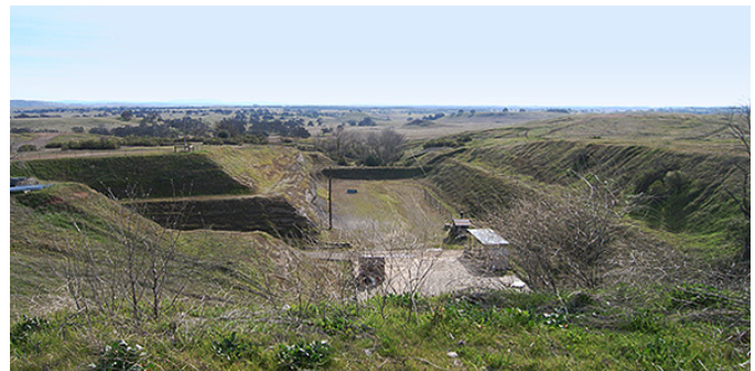
Test Stand K-1 (Aerojet Liquid Hydrogen Test Pit), now used as a shooting range.
